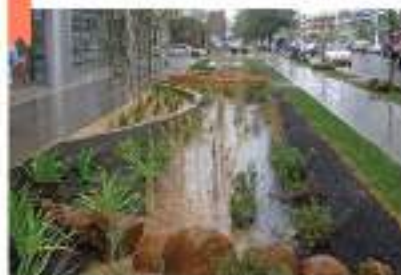
Foto di D.C. Department of Energy and Environment
